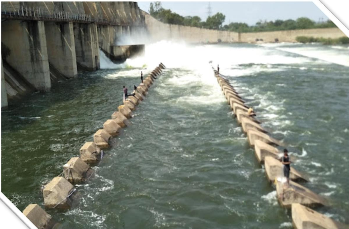
Mylavaram dam park
